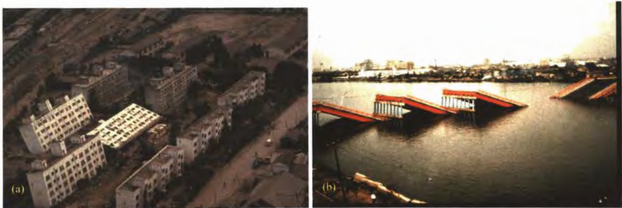
Figure 1-2a,b: Typical damage from 1964 Niigata, Japan Earthquake (a) factory (b) Shinano River Bridge ( http://www.johnmartin.com/earthquakes/eqshow/images )
