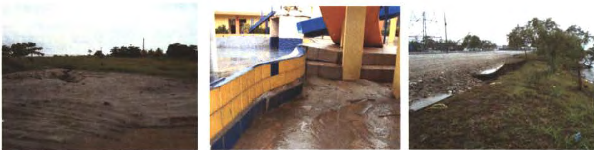
Figure 5-3: Sand boils and Lateral Spreading near Puerto Cortes and Omoa
