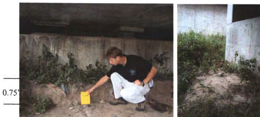
Figure 5-4: Sand boils and settlement near a bridge abutment on the Ulua River
