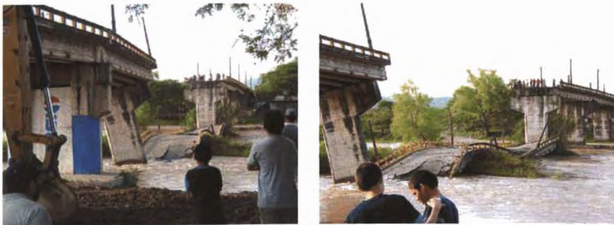
Figure 5-11: Collapsed Sections of the Humuya River Crossing (La Prensa, 2009)
